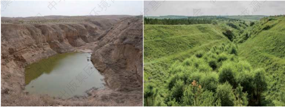
The gully(left) before reconstruction and the gully(right) after reconstruction in the project site
