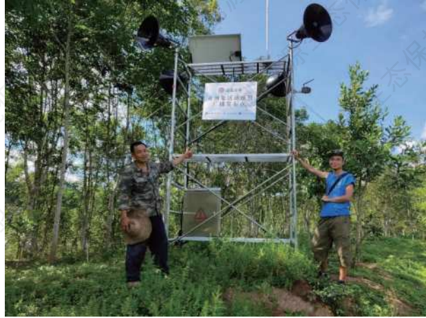
Sound-Light Warning System
