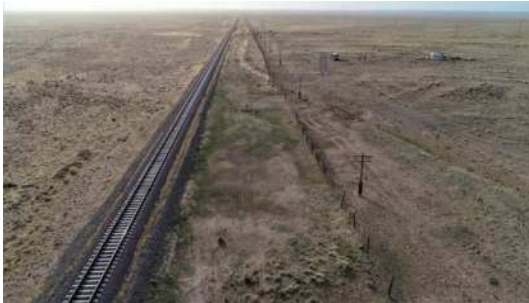
WCS Monitoring of Fence Free area
