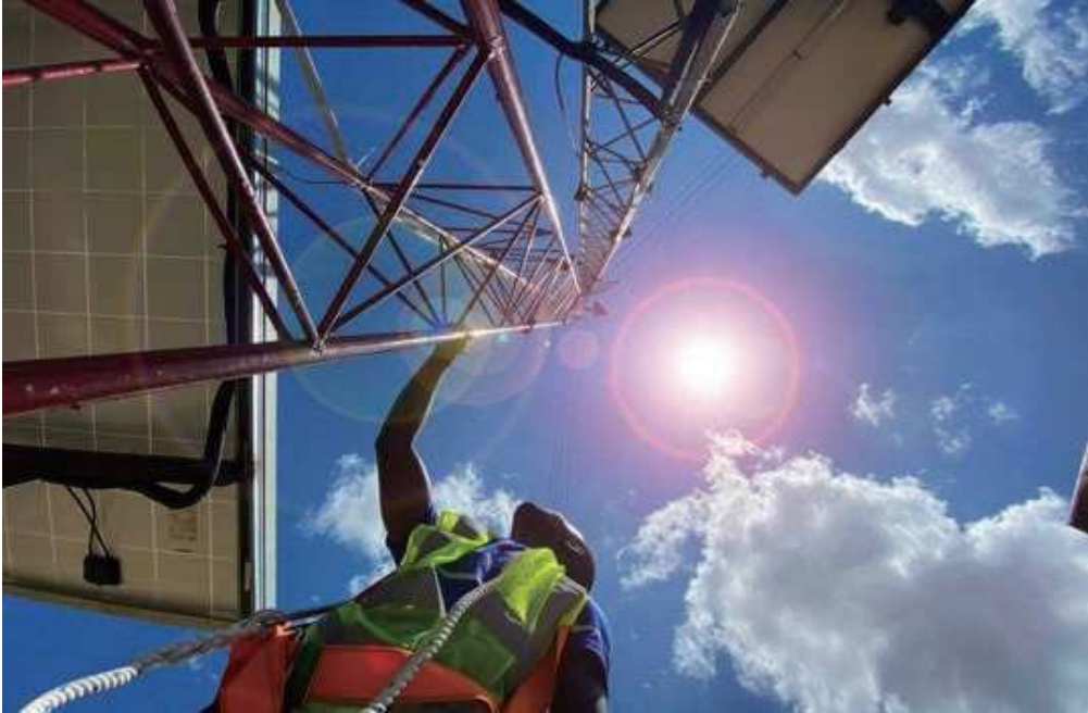
Landscape Installing enabling infrastructure for connectivity and communications
